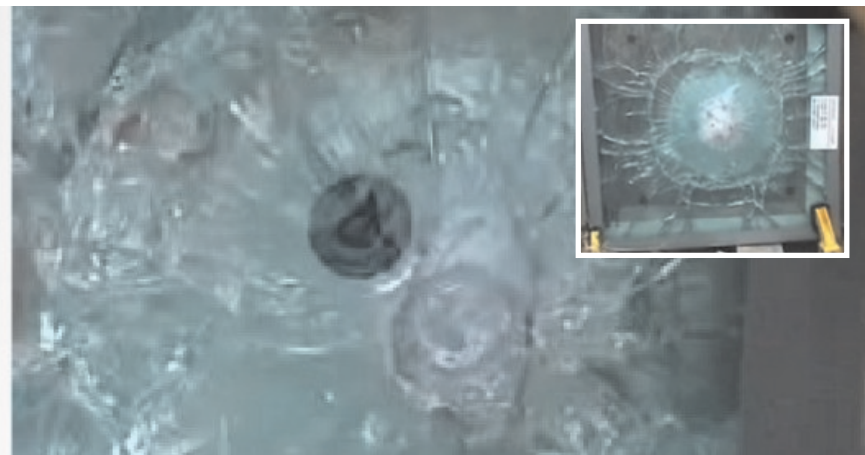
Protected window after gun shot and large object strike (inset), showing nil penetration
