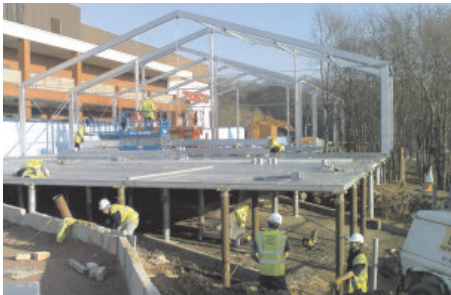
Robust, self-levelling legs core to system
